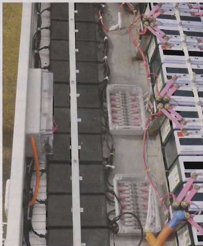
This view shows 10 of the 13 individual battery chargers.
