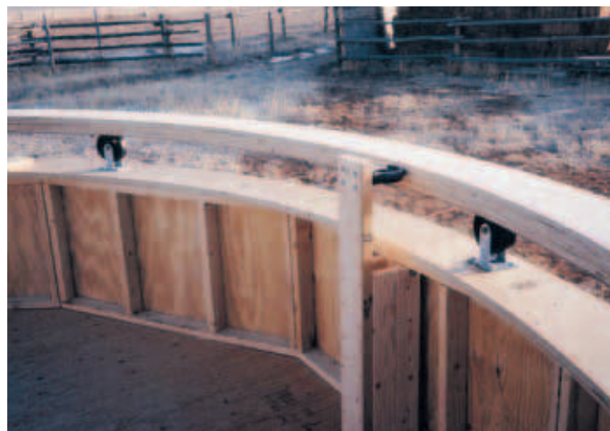
Left: MacDonald working on the observatory's 18-foot-wide, 12-sided foundation. The floor is made of 2-by-6 girders and joists and \frac{3}{4} -inch plywood, while the walls consist of 2-by-4s covered with wooden siding. The telescope's concrete pier extends to floor level. Right: The 19-foot-diameter dome and base rings made from several layers of \frac{3}{4} -inch plywood. Notice the 5-inch, heavy-duty support and guide-wheel assemblies.
