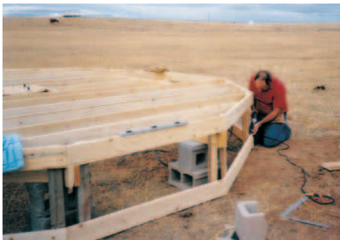
Left: MacDonald working on the observatory's 18-foot-wide, 12-sided foundation. The floor is made of 2-by-6 girders and joists and \frac{3}{4} -inch plywood, while the walls consist of 2-by-4s covered with wooden siding. The telescope's concrete pier extends to floor level. Right: The 19-foot-diameter dome and base rings made from several layers of \frac{3}{4} -inch plywood. Notice the 5-inch, heavy-duty support and guide-wheel assemblies.
