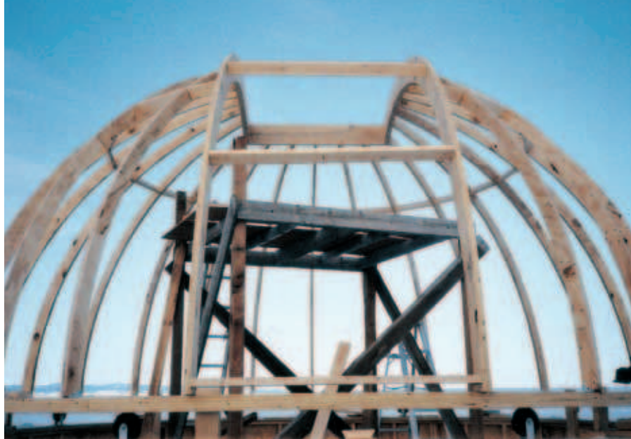
The completed dome framework with all 21 ribs fastened to the nearly 5-foot-wide slit frame. The slit extends 2\frac{1}{2} feet past overhead to allow telescope access to the zenith. The 2-by-4 crossbraces in the dome opening were removed after the dome skin was attached.
