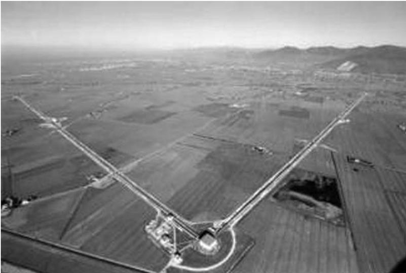
FIGURE 6.4 The VIRGO interferometer located at Cascina, in the countryside near Pisa. The picture – taken from a plane – shows an aerial view of the current interferometric configuration. The two arms (3 km long, oriented at 90 degrees to one another) contain the vacuum pipes within which the laser beam is transmitted. (Picture courtesy of the VIRGO collaboration)
