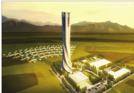
Tracking the Sun China's 1.5 MW Dahan solar-thermal plant will use 100 mirrors to focus the Sun's light to generate electricity.
